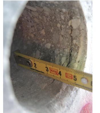
stable delamination (no spalling)
